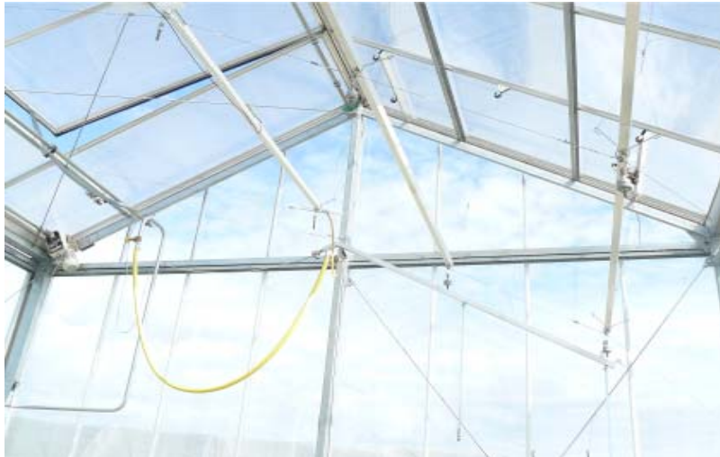
Fig. 5. The three collectors of the system inside the greenhouse, with details of the suspension and steering construction of the solar cell modules.
