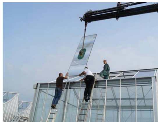
Fig. 3. Placement of the three Fresnel lenses of 1 \times 1 m between double glass (size of 1 \times 3 m).
