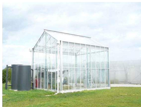
Fig. 4. The Fresnel greenhouse in Wageningen at the real size of 6 \times 6 m.
