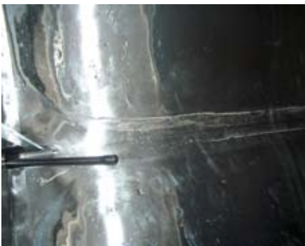
Bezinsel in tank na reiniging: links is uitstroomopening op bodem tank.
