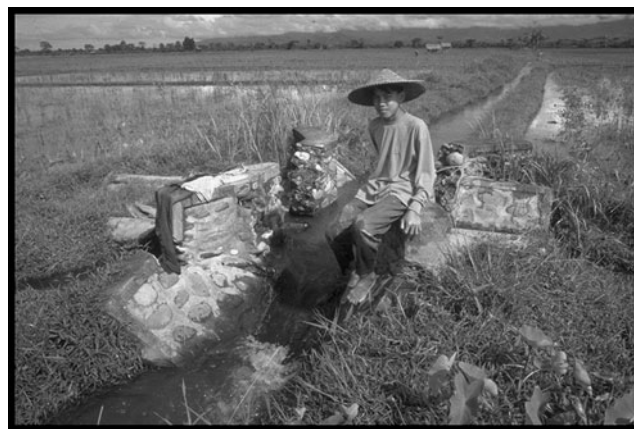
Fig. 4 Degraded TU infrastructure (photo by author)
