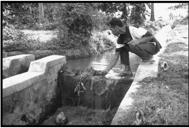
Fig. 5 Farmer-constructed temuku (photo by author)
