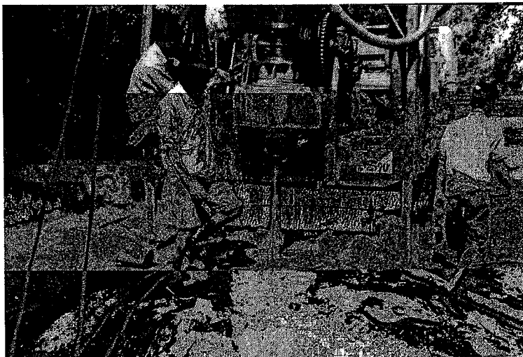
PICTURE 4.1: INSTALLATION OF A TUBEWELL
