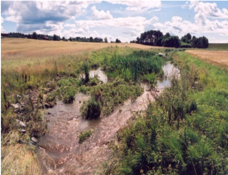
Photo 12.6 Example of a constructed wetland in Norway
