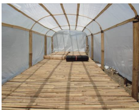
Figure 4. Inside details of the nursery construction.
