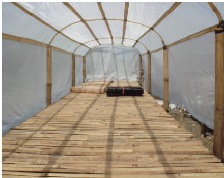
Figure 4. Inside details of the nursery construction.
