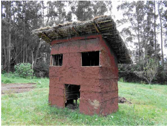
Picture 5.2.3: Example of a ware potato storage at Holetta Agricultural Research Center. The wide roof provides shade on the walls, so the inside temperature stays low.
