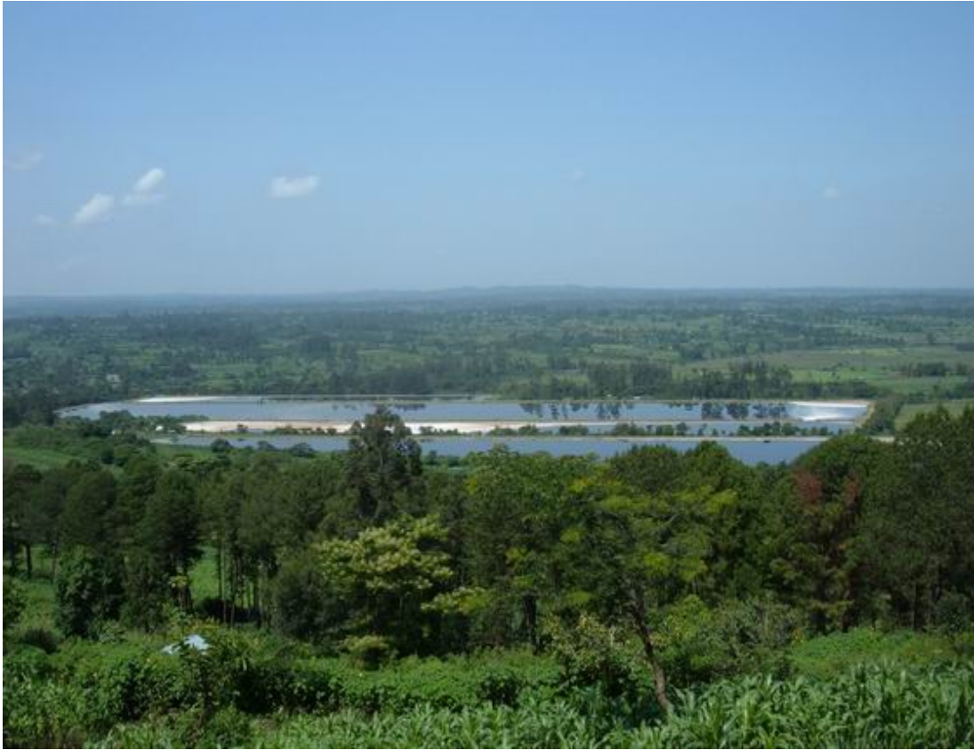
Fig 2.2 A view of PANPAPER Mills wastewater treatment ponds
