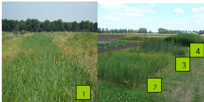
Fig. 1 Surface flow wetland (left) and three field scale constructed wetlands (right). Numbers refer to table 1
