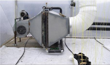
*An early version of an ATU in the 1990s in New Zealand: air is heated by hot water pipes and then spread through air ducts.*
