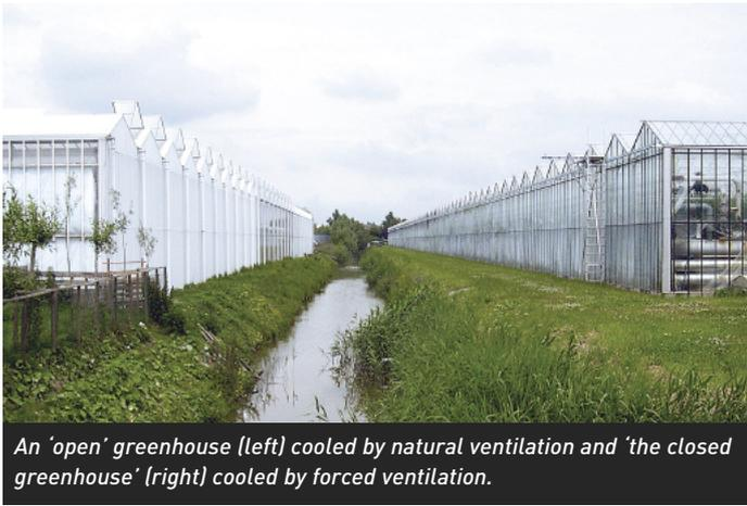
An 'open' greenhouse (left) cooled by natural ventilation and 'the closed greenhouse' (right) cooled by forced ventilation.
