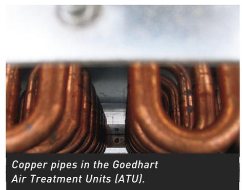
*Copper pipes in the Goedhart Air Treatment Units (ATU).*
