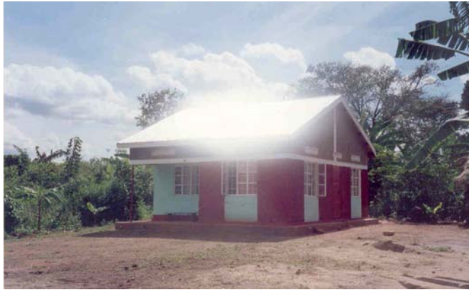
A simple house constructed by the World Vision Office for a needy household in Kasawo sub county
