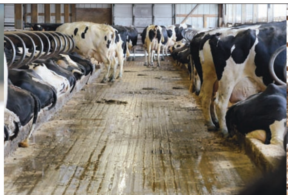
The passageways are too narrow
