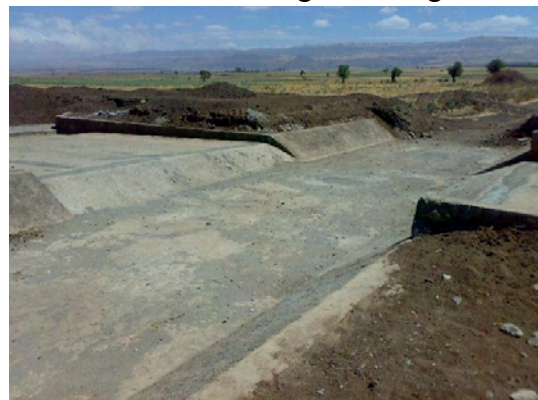
Figure 4.5: Cross level structure at main canal before branch canal 2
