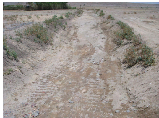
Figure 4.10: Observation of the canals
