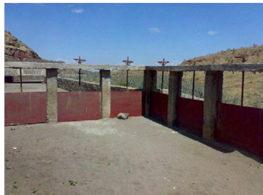
Figure 4.4: The sluices and rejection spillway
