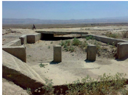
Figure 4.9: Sedimentation at division box
