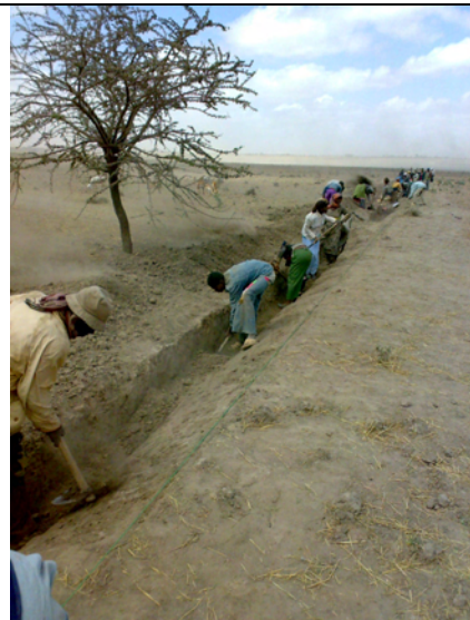
Figure 4.11: Preparing a tertiary canal
