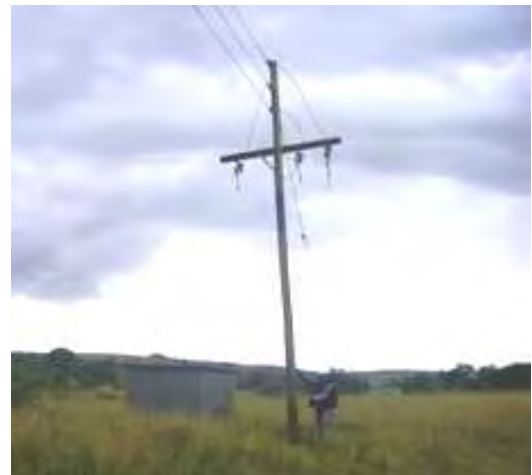
Picture 6.19: Missing transformer at groundwater pump
