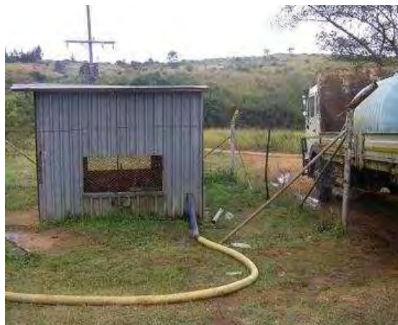
Picture 6.18: Water abstraction from borehole
