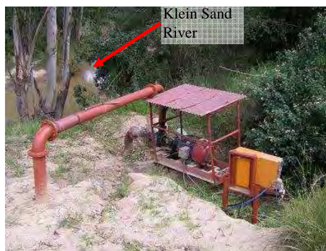
Picture 6.7: Abstraction pump at Klein Sand River Source: author, 2009
