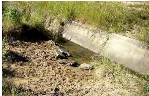
Picture 6.12: Broken main canal at Dingleydale, due to cattle crossing Source: author, 2009
