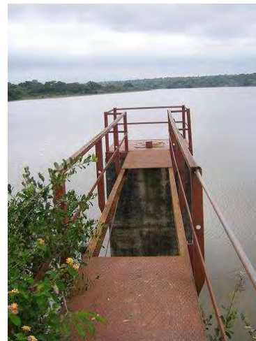
Picture 6.16: Missing steel plates at outlet tower Orinoco dam
