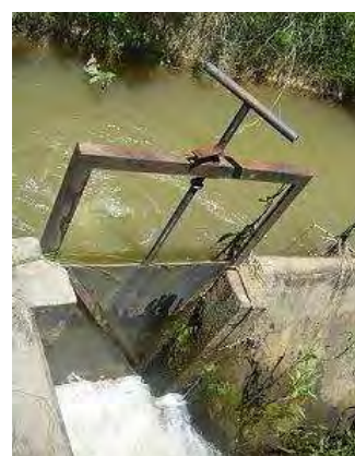
Picture 6.2: Broken gate at Dingleydale
