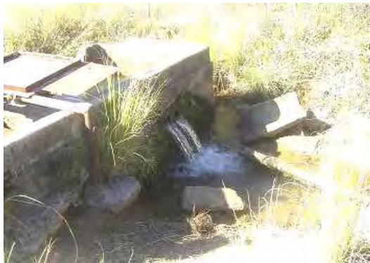
Picture 6.13: Broken secondary canal at New Forest Source: author, 2009
