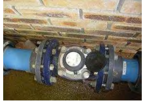
Picture 7.1: Non functioning flow meter at Zoeknag water treatment plant
