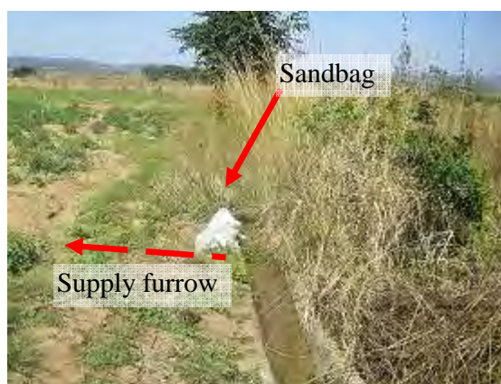
Picture 6.15: Secondary canal with sandbag
