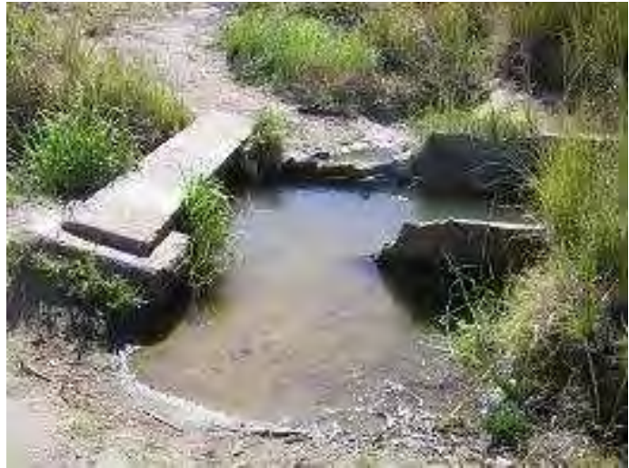
Picture 8.3: Broken section of Dingleydale main canal Source: Author, 2009
