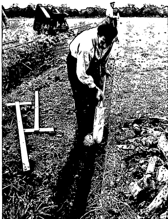
Figure 1. Subsurface drain installation by hand (1952). (By courtesy of Government Service for Land and Water Use).
