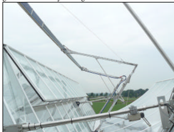
Fig. 10 Side view of the framework with two linear actuators and the PV cells.
