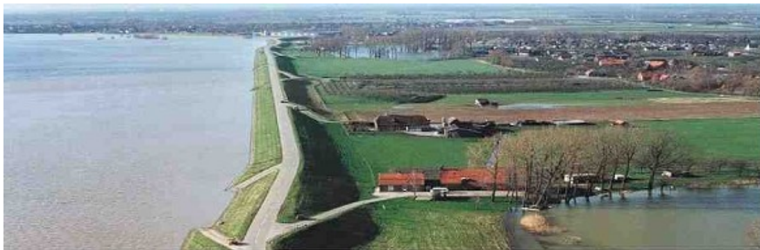
Figure 5: The water level on the river is rising.
