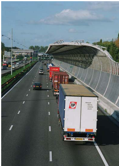
Fig. 6. Acoustic shielding used for compartmentalization.
