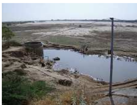
Figure 4.3 Banas River: water storage behind underground dam
