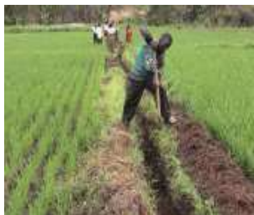
Photo 5.1 A man clearing a tertiary canal to allow more water for rice plots
