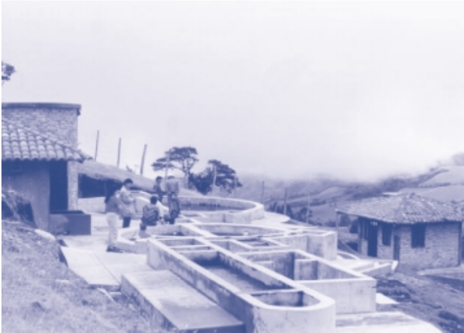
Figure 5. Photo of the MSF plant (SSF + pre-treatment) in Paispamba, Colombia
