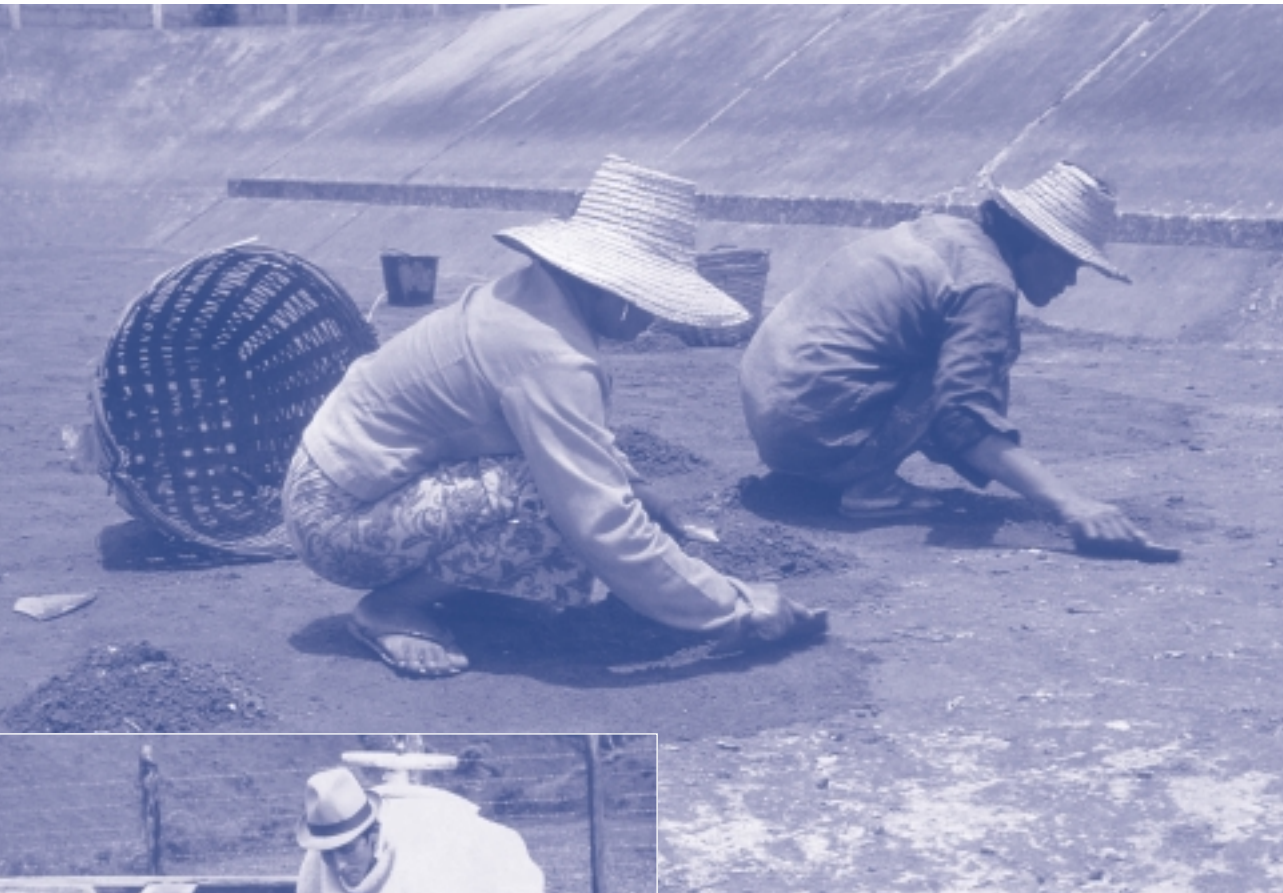
Operators at work on slow sand filters.
