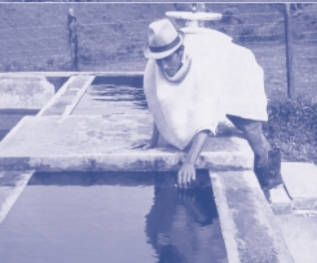
Operators at work on slow sand filters.
