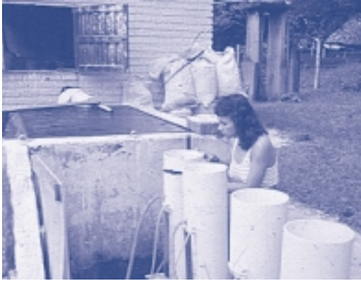
Figure 12. A pilot plant for pre-treatment research in El Retiro, Colombia
