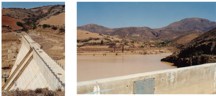
Figure 3.8 General views of the Laka-Laka dam and reservoir
