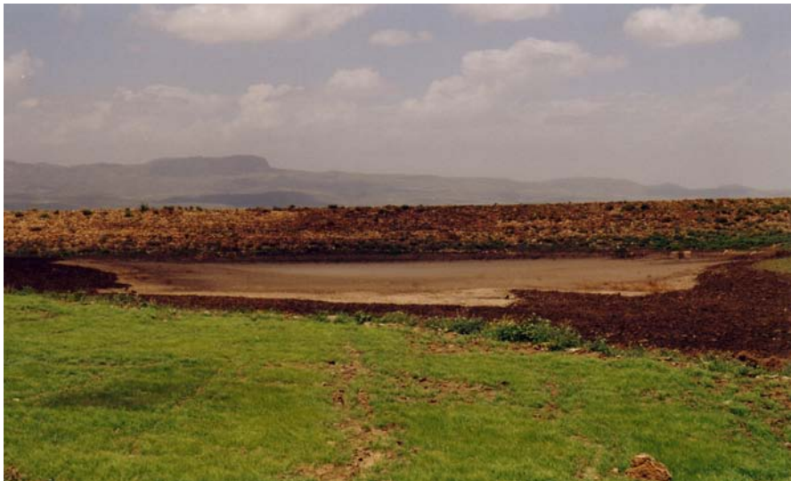
Figure 7.2 Mejae reservoir totally silted up by sediment (Poesen, et al. , 2001)
