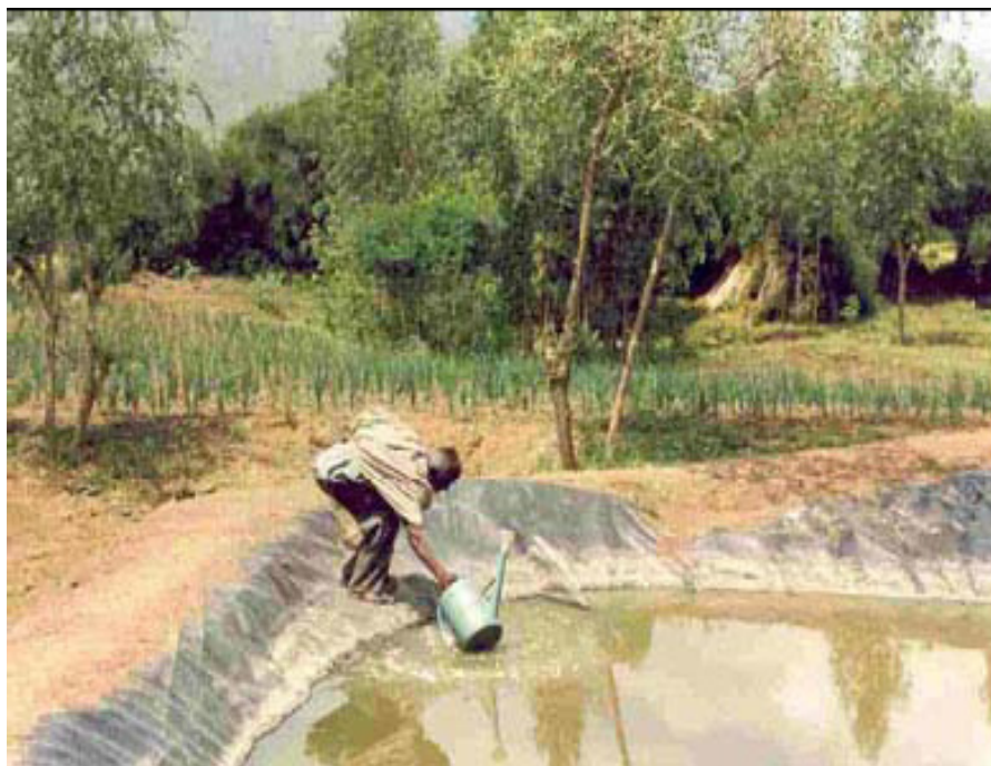
Figure 3.12 Farmer fetching water from his plastic lined pond in Alamata, Tigray (Rämi, 2003)
