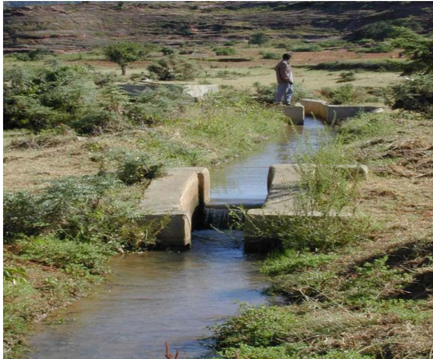
Figure 3.11 Partial view of irrigation canal being used in Tigray
