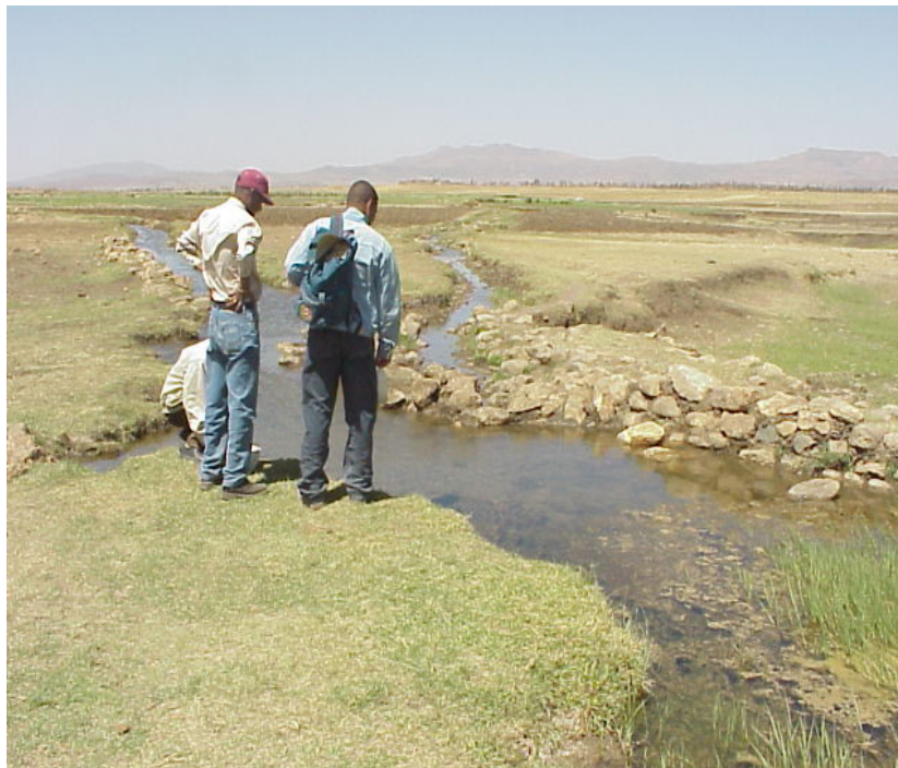
Figure 6.8 Temporary seepage diversion structure at Gumsalasa
