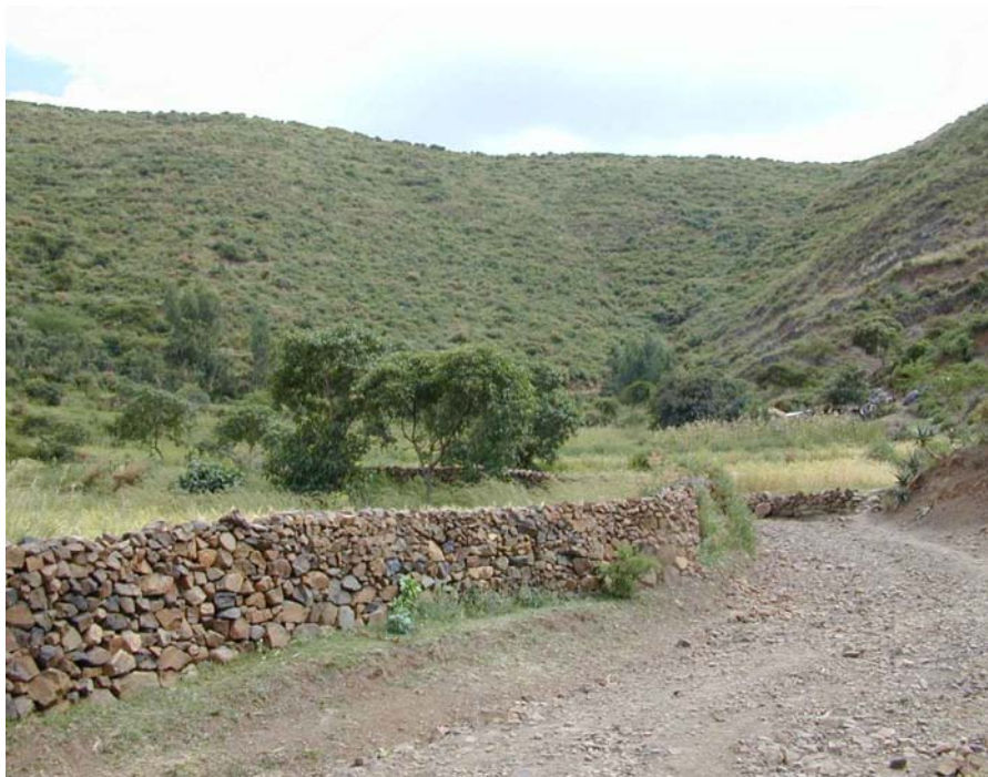
Figure 3.8 View of the catchment area, the stone-faced trenches and natural regeneration in one of the earthen dam irrigation schemes
