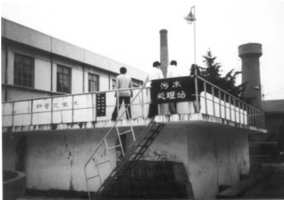
Photograph 6.6 Wastewater treatment station of Hengshanqiao Woolen Mill No. 8
