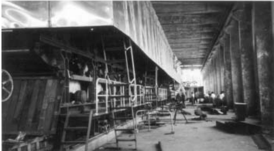
Photograph 7.3 Yuejin paper mill under renovation
