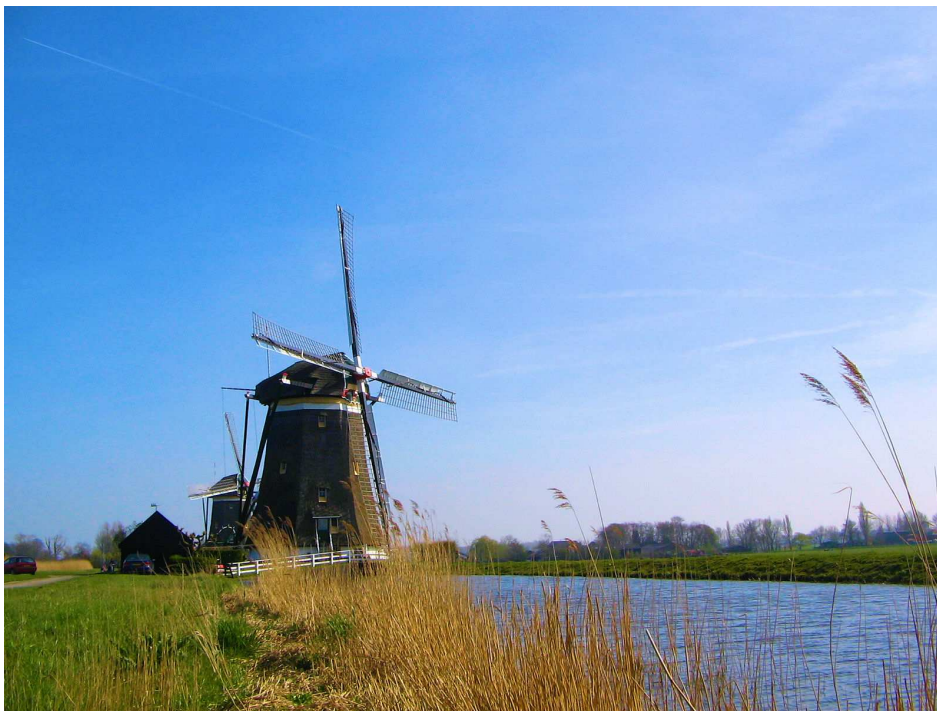
Figure 4: The traditional Dutch polders were made with the help of wind energy: the windmills pumped up the water into the canal system, sometimes in a series such as here at Stompwijk, when the difference was too much for one windmill. As a result, much of the land is below the present-day sea level. Nowadays the land is kept dry by modern pumps. Photo: Sander Klaver.
